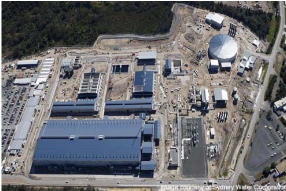
Figure 1: The Sydney Plant (Courtesy of Sydney Water)
