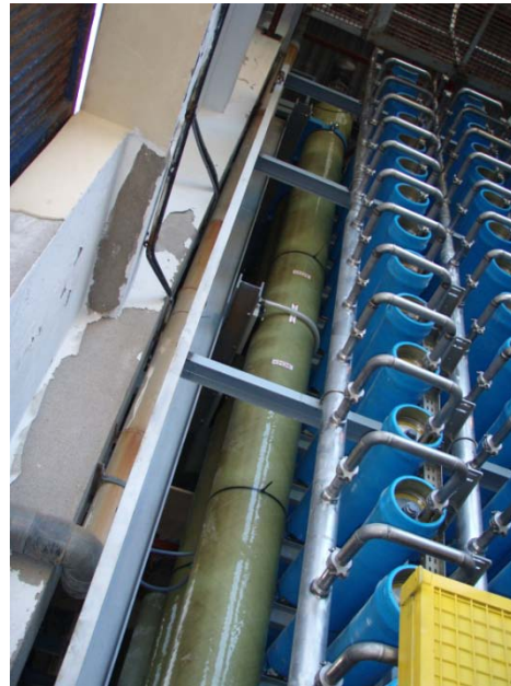
Figure 3: Las Palmas FRP vessel
