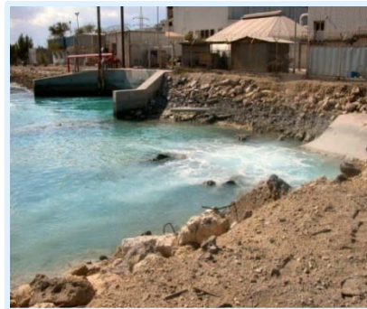
SPWS/ phase I&III outfalls
