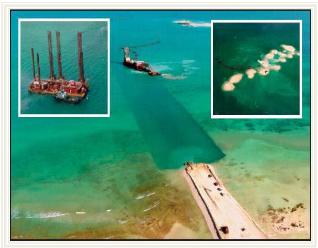
Figure 5: Dredging and blasting during construction of Raf B
