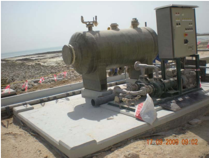
Figure 15: Vacuum tank and pump skid
