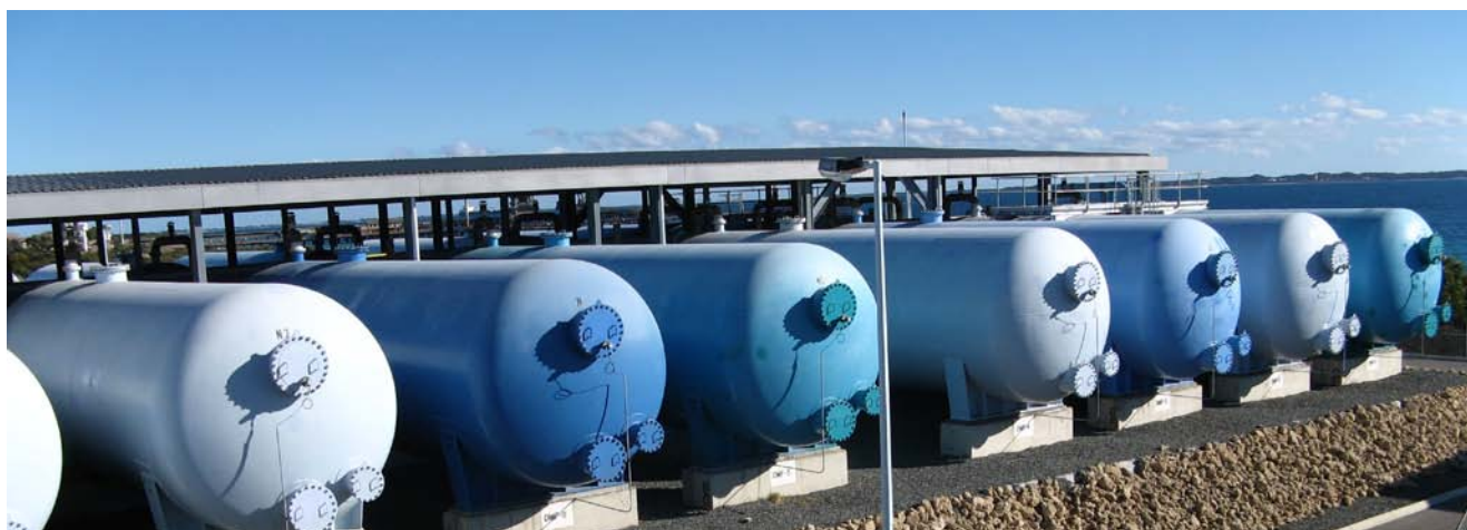
Photo 11: Dual Media Filters of the PSDP
