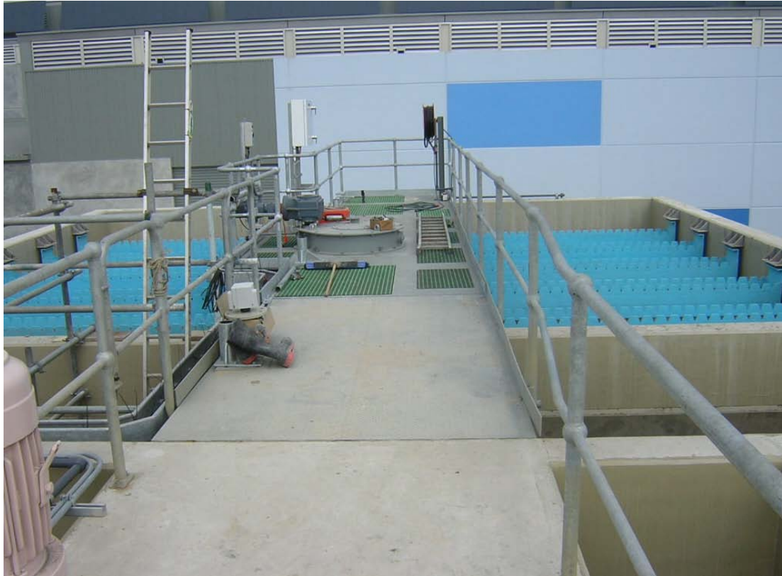
Photo 12: 'Densadeg' – Clarifier of backwash waste water
